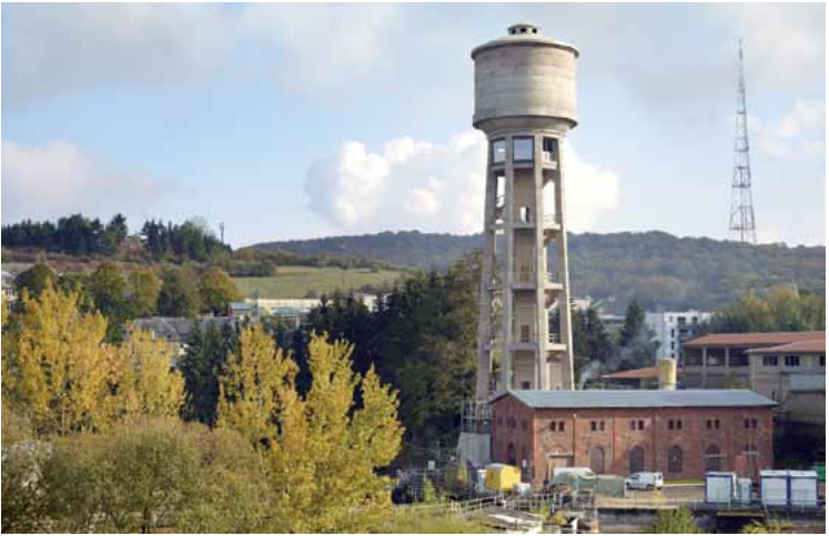
Wasserturm &amp; Pumpstation, Dudelange
